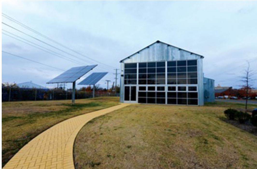
Scott Elmquist A paved, yellow-brick sidewalk leads to a former metal trolley car barn on Brook Road in North Side that was restored to serve as offices for Dovetail Construction.
