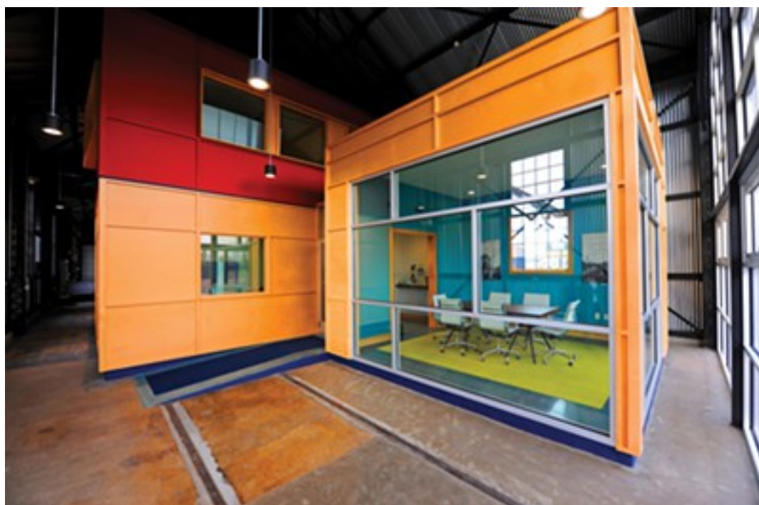
Scott Elmquist A colorful, boxlike addition was inserted in the historic structure and is heated and cooled by geo-thermal wells.
