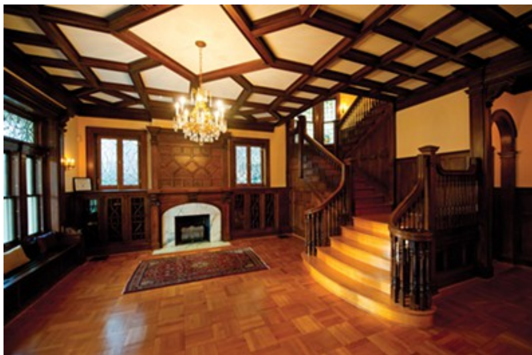
Scott Elmquist All of the interior surfaces, including the side paneling, fireplace, coffered ceiling and parquet floors of the stair hall at 2710 Monument Ave. were refinished.
